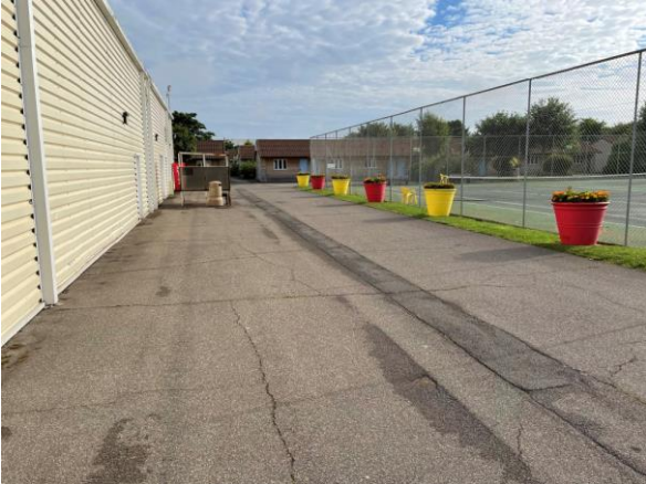
4.1 Existing macadam along east elevation of premises
