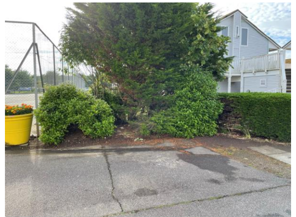
4.4 SW corner of tennis courts, soft landscape will be retained in these locations
