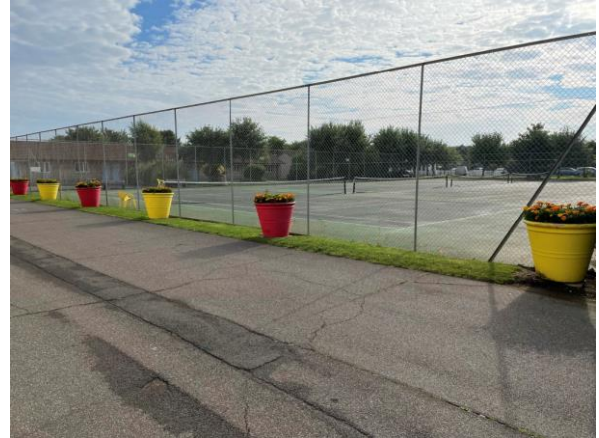
4.2 Existing tennis Courts and Fencing on east elevation of premises
