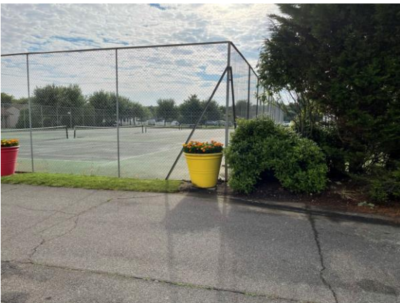
4.3 Existing tennis courts and fencing at southwest access point of play equipment
